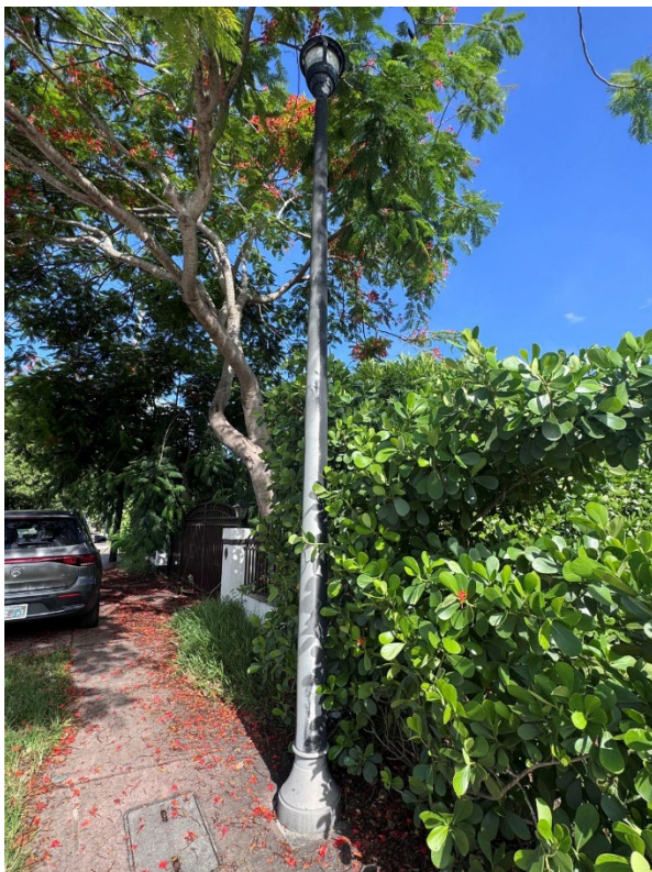
Worn and missing paint
