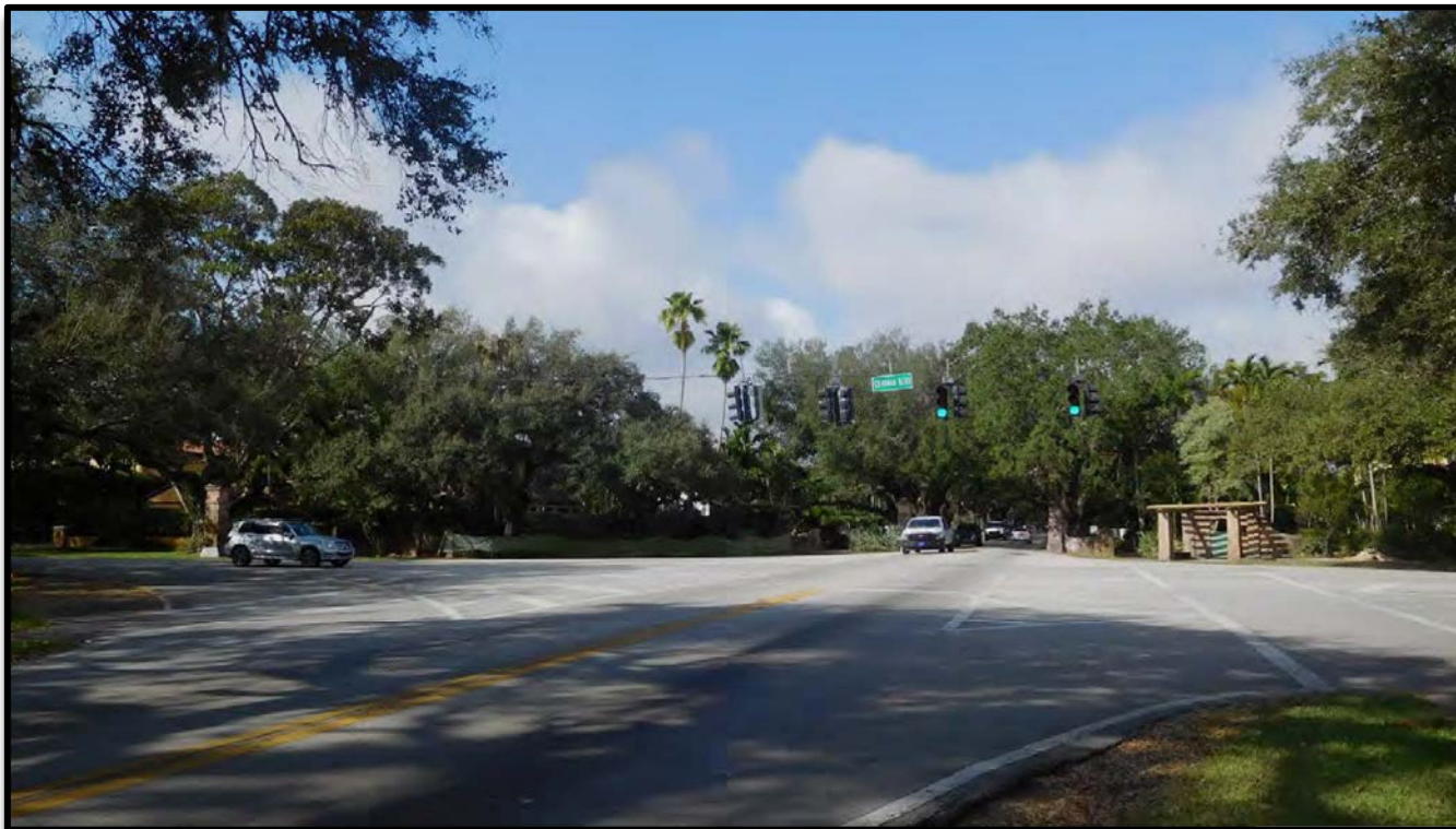
Coral Way and Granada Boulevard – Existing Condition
