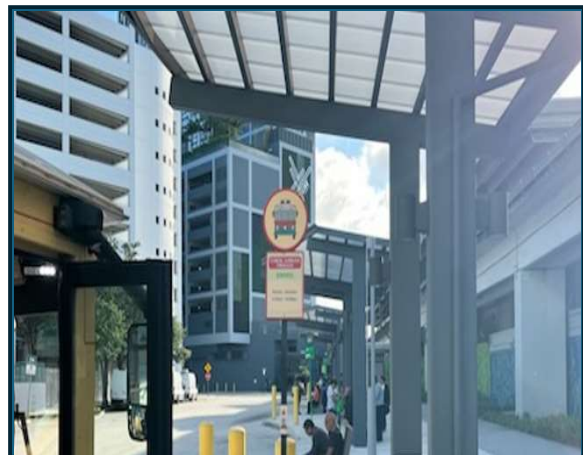
Douglas Road Metrorail Station
