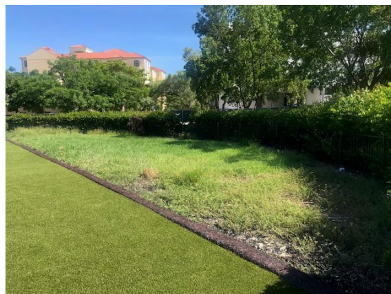
Image 12. Potential drainage concern with standing water remaining behind unitary rubberized curbing. Drainage holes were added to the border surrounding the artificial turf safety surfacing but should be tested for standing water during next heavy rainfall. Standing water may affect the impact attenuation of the safety surfacing.
