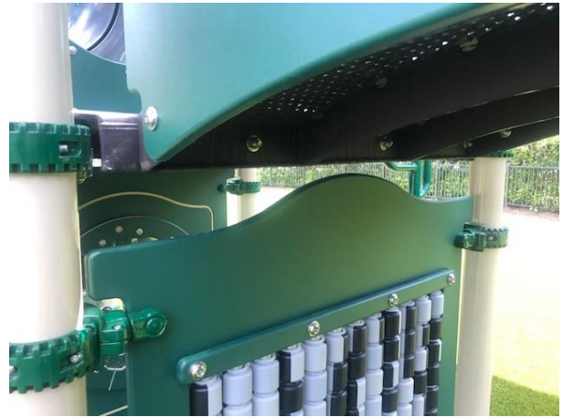
Image 9. Potential head entrapment hazard on bottom play panel – gap exceeds 3.5in on either side and is enclosed by support posts
