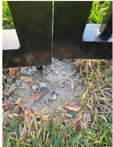
Image 5. Service entrance missing sleeve for gate peg.
