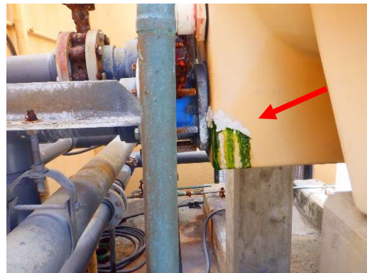
Crack Bottom of Chiller Housing
