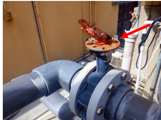
Corroded Water Valves
