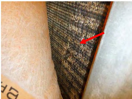
Brittle Heat Pump Coils
