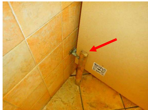
Bathroom Partition Not Secured
