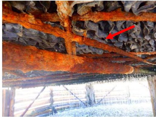
Corroded Pipe and Frame
