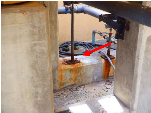
Corroded Pipe Hangers
