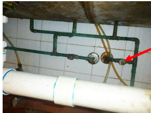
Missing Stem Valve Handles
