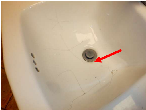
Cracked Bathroom Sink
