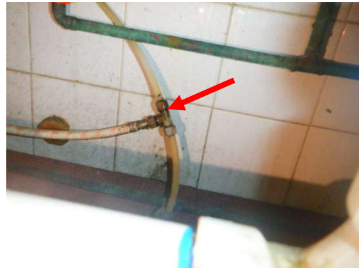
Water Leak Below Sink
