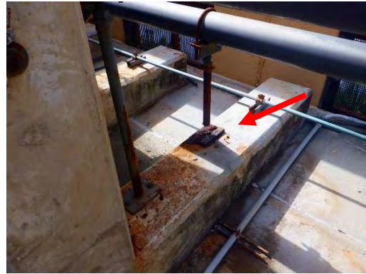
Corroded Pipe Stands
