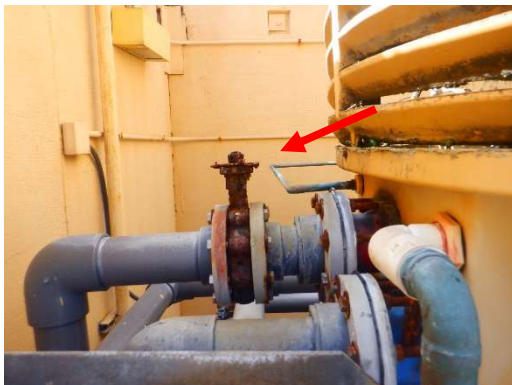
Corroded Valve Handles
