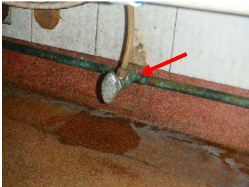
Water Leak Below Sink
